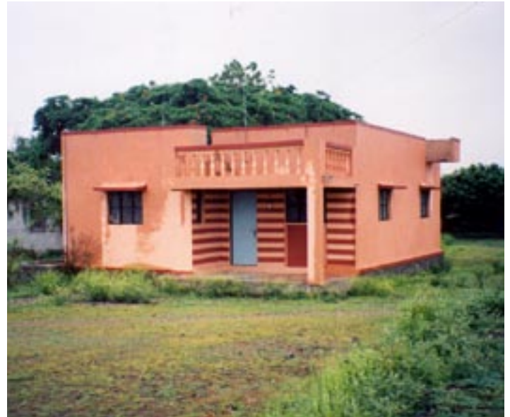
Pumpkin House India will begin operations in this rented home in Vidyanagar, a community near Meherabad, India.
